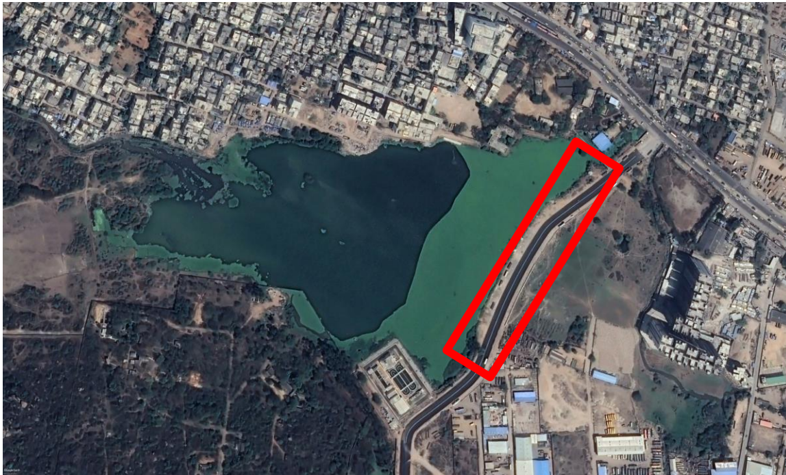
April 2014 – Newly constructed wide metalled road
