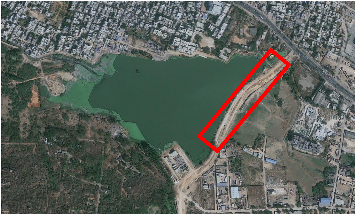
January 2012 – Road construction work started.
