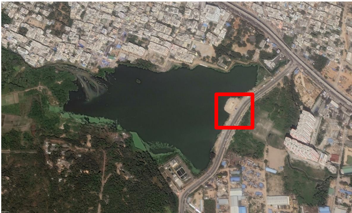
November 2016 – Immersion Pond construction started
