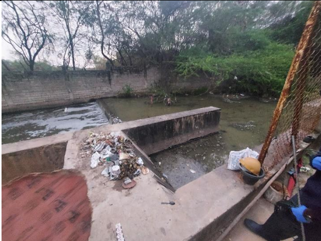
Figure 9: This image shows Point 2 demarcated on Figure 1 (Identified as the STP inlet). Point measurements were undertaken for eight points on an hourly basis.
