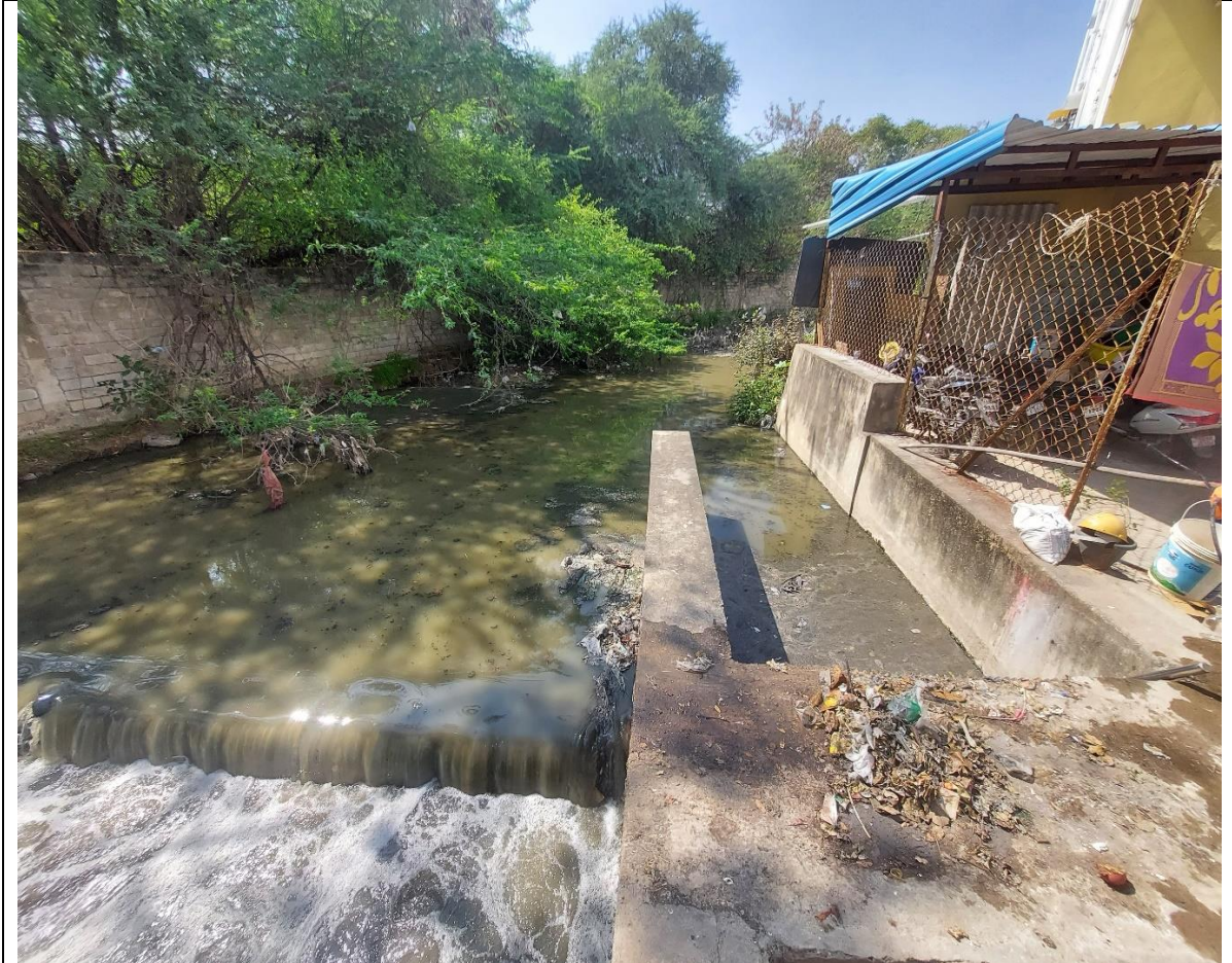
Figure 13: Water diversion structure at Balajinagar (Sample Point 2a and 2b) – The channel on the left carries water directly into the lake and the one on the right screens solid waste and conveys water to the pumping station
