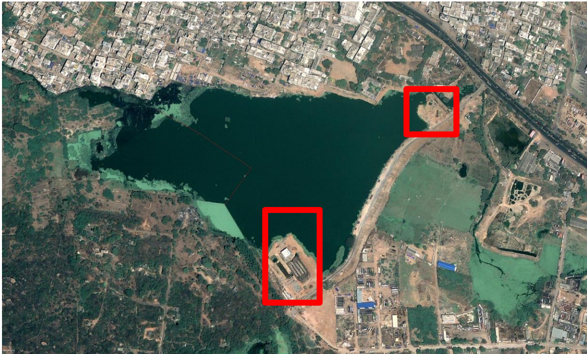
February 2010 – construction of STP and pump house
