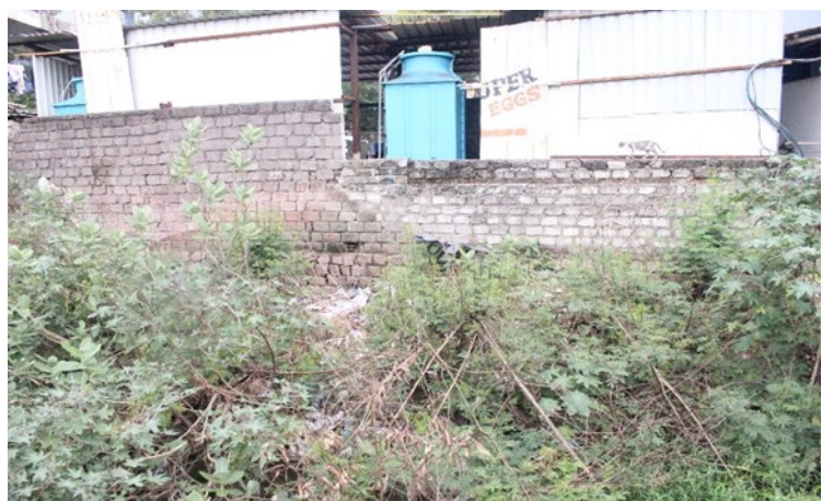
Encroachments on lakebed
