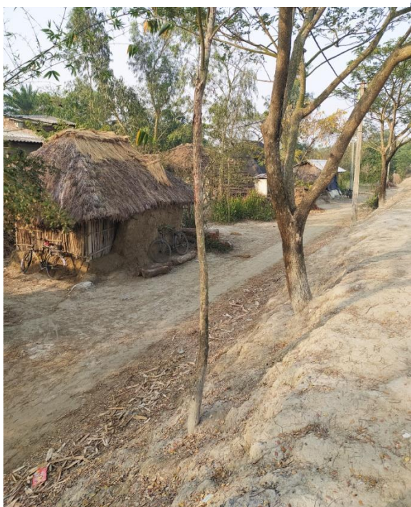
Photo 4.10: Kuchha mud housing with straw roof adjacent to earth embankment in Gosaba block
