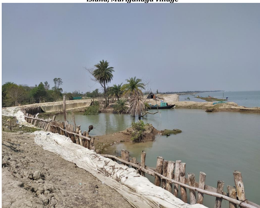
Photo 4.7: Ring embankment constructed after embankment breach and land erosion/loss on Sagar island, Muriganaga village
