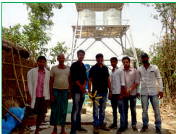
Figure 5. Installation of Arsenic Filter
