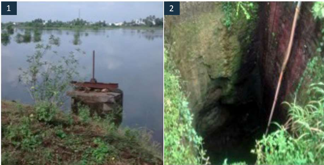
Picture 1: Sluice and water spread area of non-system tank
