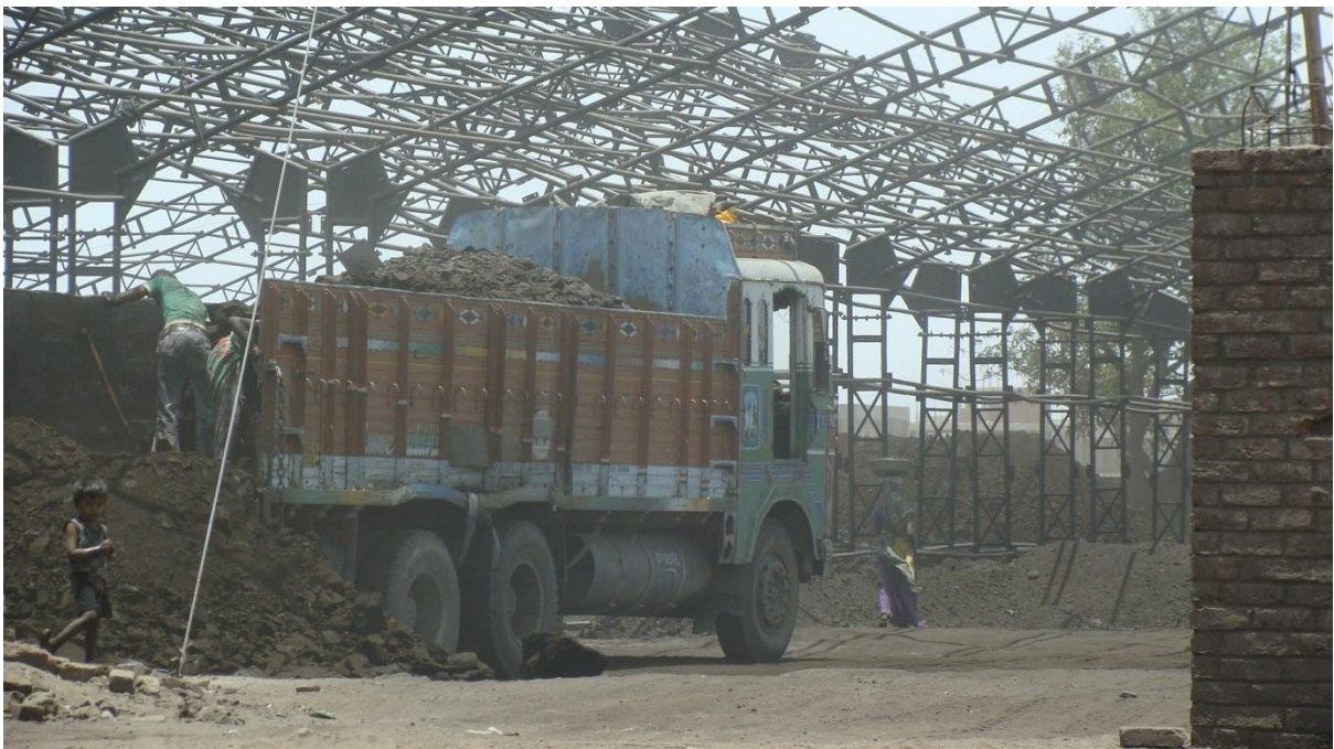
Concrete mixing is being done in this plant
