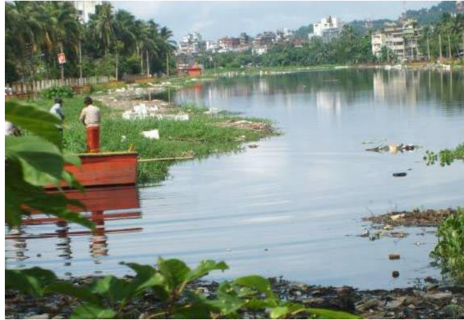
Open drains in the peri urban Guwahati
