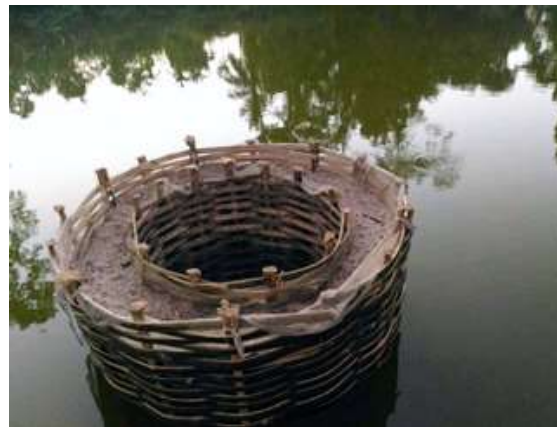
Household level Pond water based filter Alternative source for Drinking water Titabar, Jorhat (Assam)
